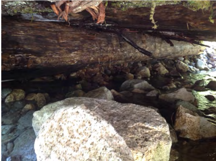
Left Bank Abutment when facing downstream
