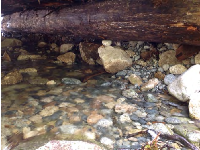
Left Bank Abutment when facing downstream
