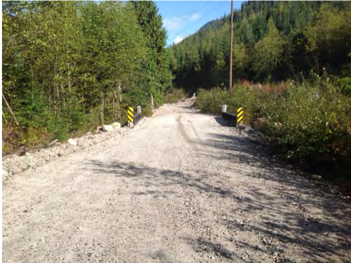
Approach from Left Bank when facing downstream
