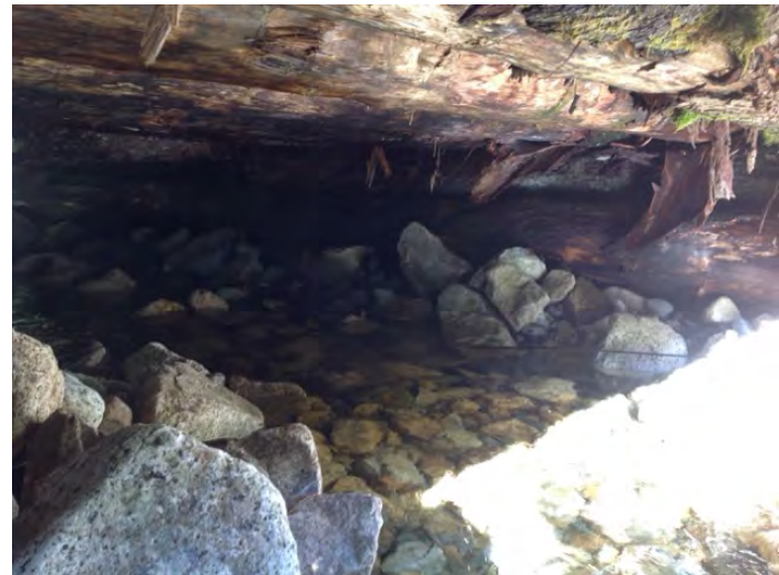
Right Bank Abutment when facing downstream
