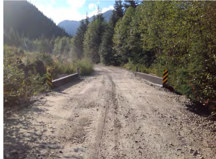
Approach from Right Bank when facing downstream
